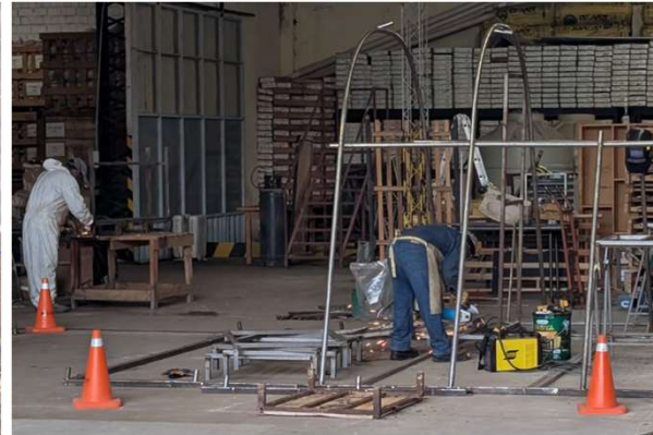
Centauri workers refurbishing camp facilities for Rio Grande project
